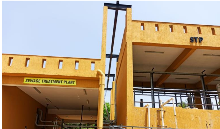
SEWAGE TREATMENT PLANT
