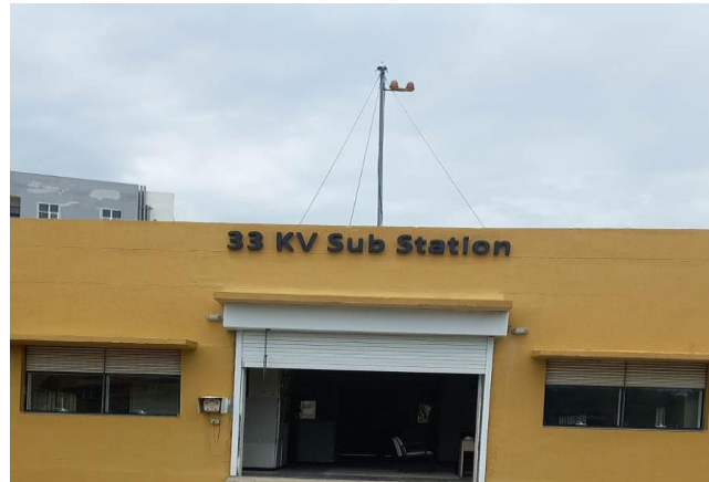
33KV Sub Station
