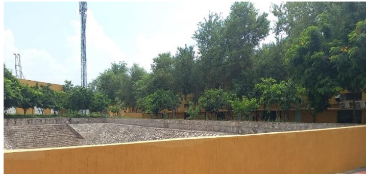
Rainwater Harvesting Yard
